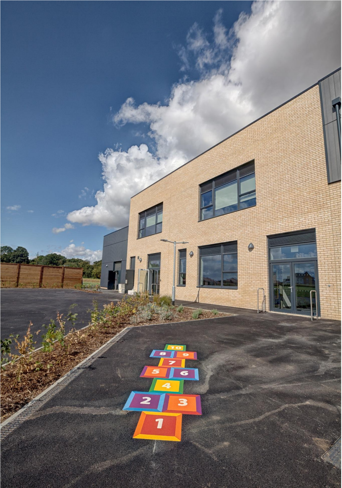
Limebrook Way Primary School, Maldon (rear view)
