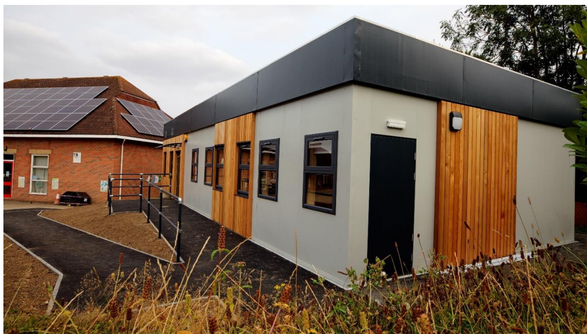
Cold Norton Primary School, Cold Norton (double classroom block)
