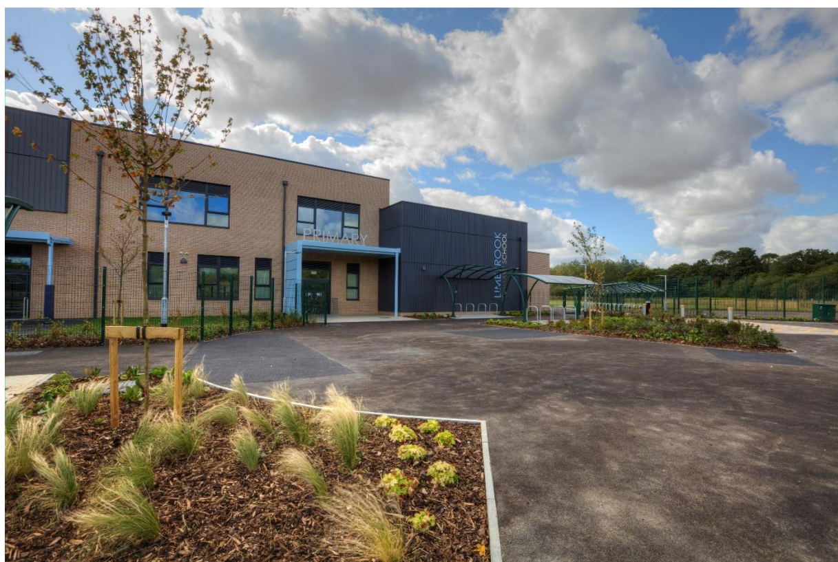
Limebrook Way Primary School, Maldon (main entrance)
